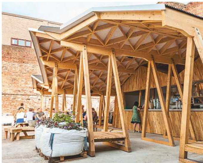
Constellations Bar by Hugh Miller Furniture – the canopy and all other components were prefabricated in the workshop and erected onsite in three days
